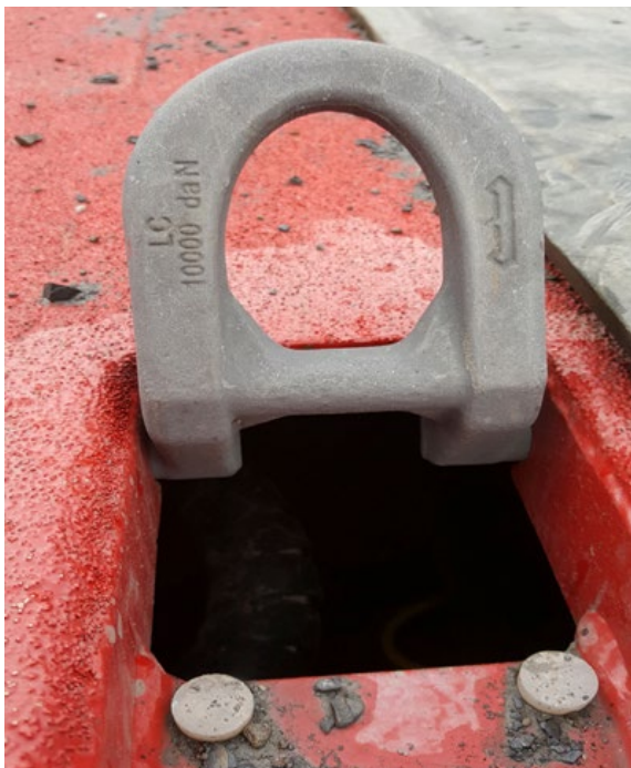
Example of anchorage point
