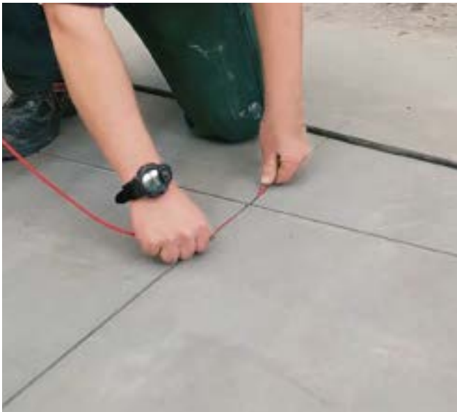
Fig. 13 Inserting the cable.
