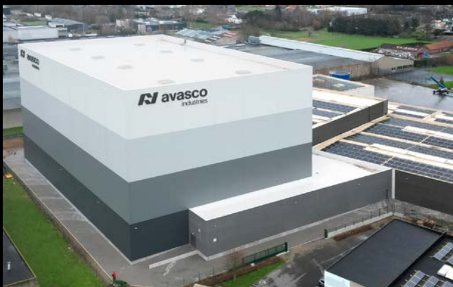
Avasco's new high-bay warehouse.
