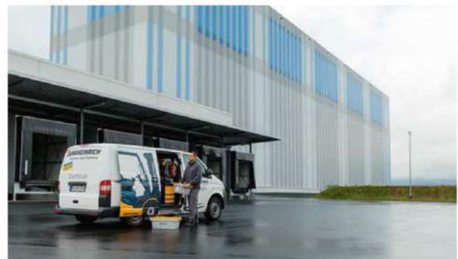
Automatic pallet high-bay warehouse, Sauer GmbH & Co. KG, Föritz, Germany.
